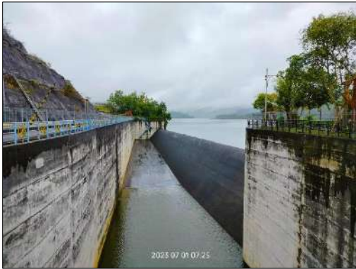
Up stream Spillway
