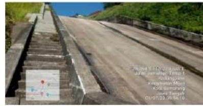
Down stream Spillway
