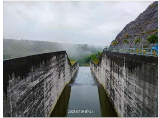
Down stream Spillway
