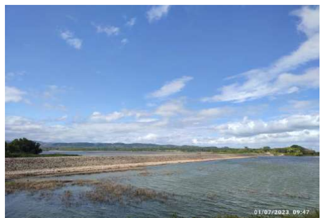
CLOSURE DIKE A
