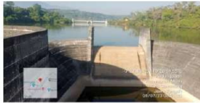
Up stream Spillway
