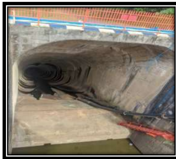
TEROWONG OUTLET SPILLWAY
